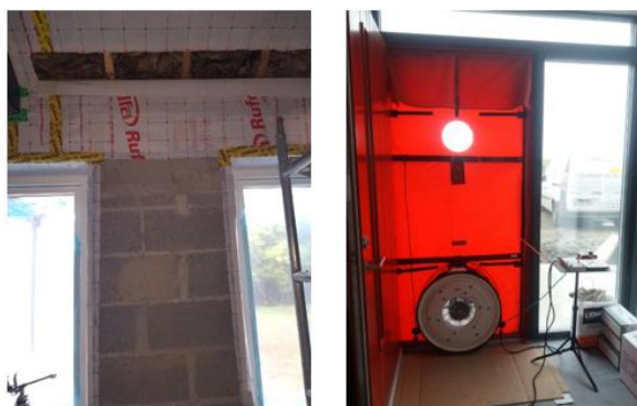
Figure 3: Air Tightness Testing
